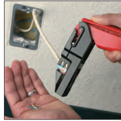
6. Wires will be seated and cut for a solid termination.
